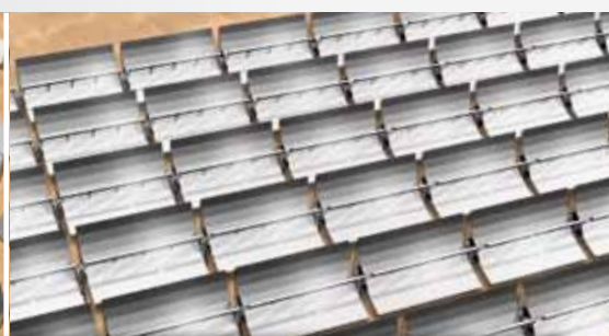
Parabolic Trough Technology
